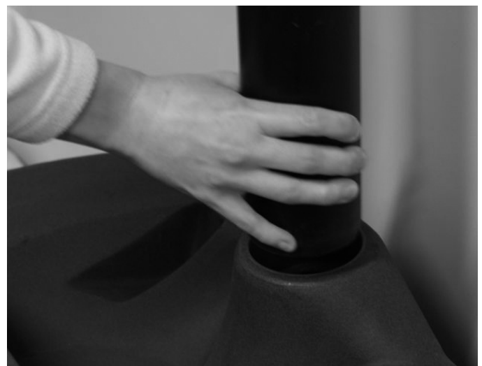
3. Disconnecting the ventilation pipe.
